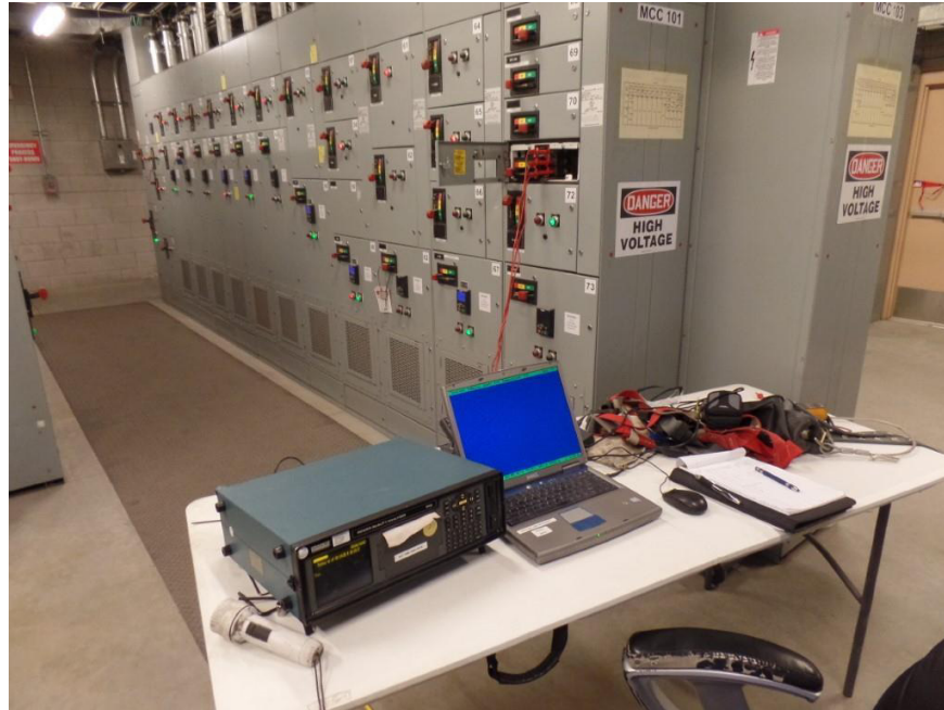
Test Set =up on Spare Disconnect in Can #71
