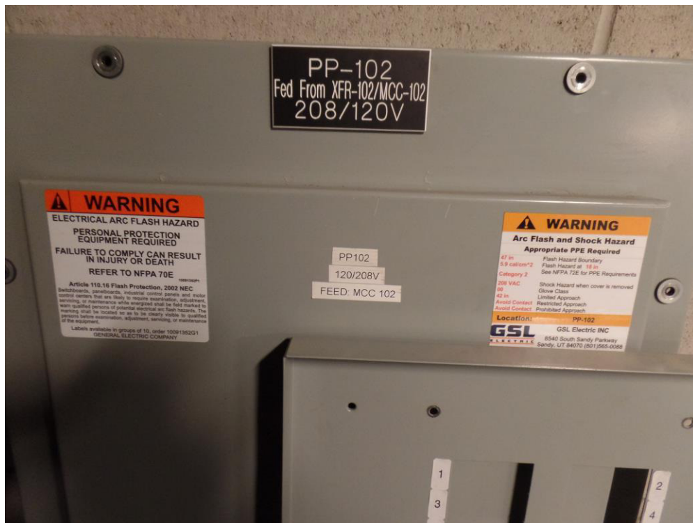
Names Plates for Power Panel PP-102
