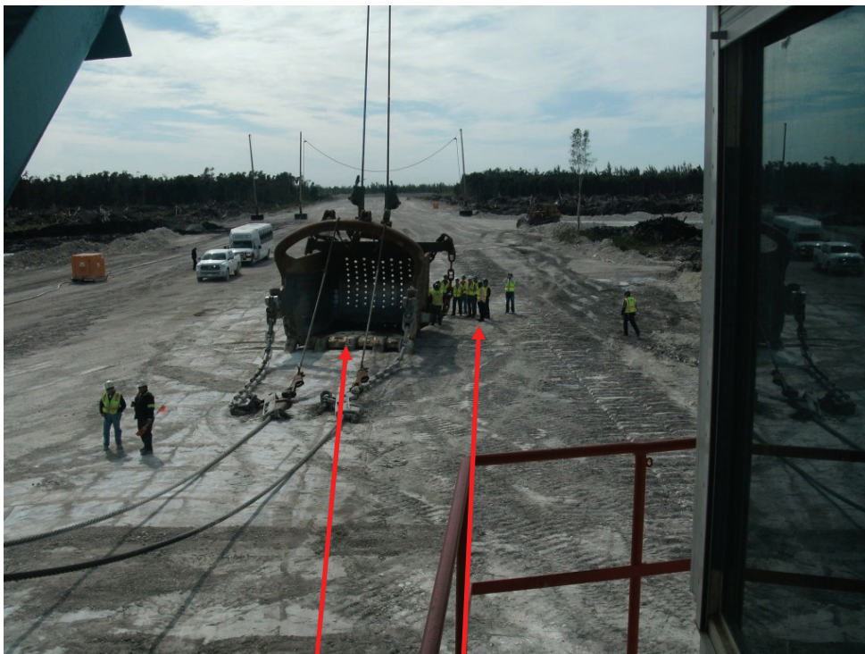
Crane Bucket (note size of people standing next to bucket)
