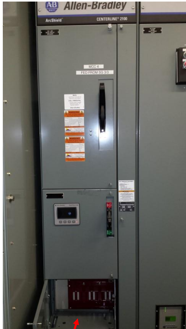
Open bucket in 3 rd slot of panel
